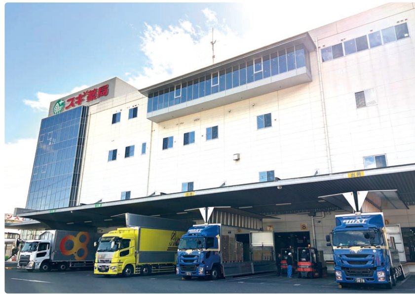
Chief distribution center attached to the Chubu Head Office
